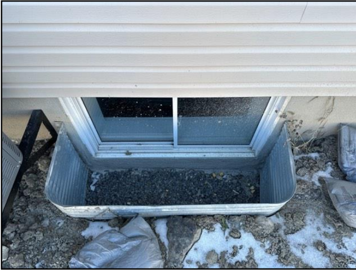
88. Clean window well
