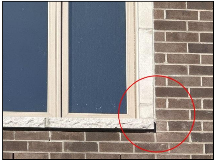
46. Masonry deterioration
