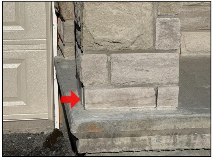
32. Masonry deterioration
