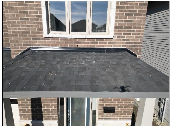
5. Remove all loose debris from roof coverings.
