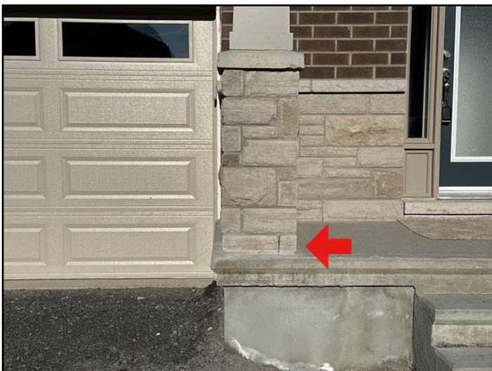
29. Masonry deterioration
