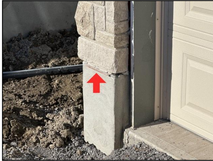
38. Masonry deterioration
