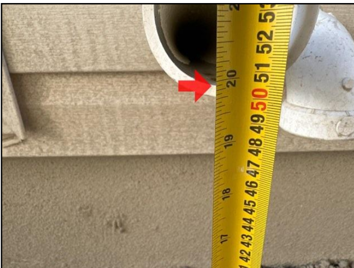
144. Clearance to grade
