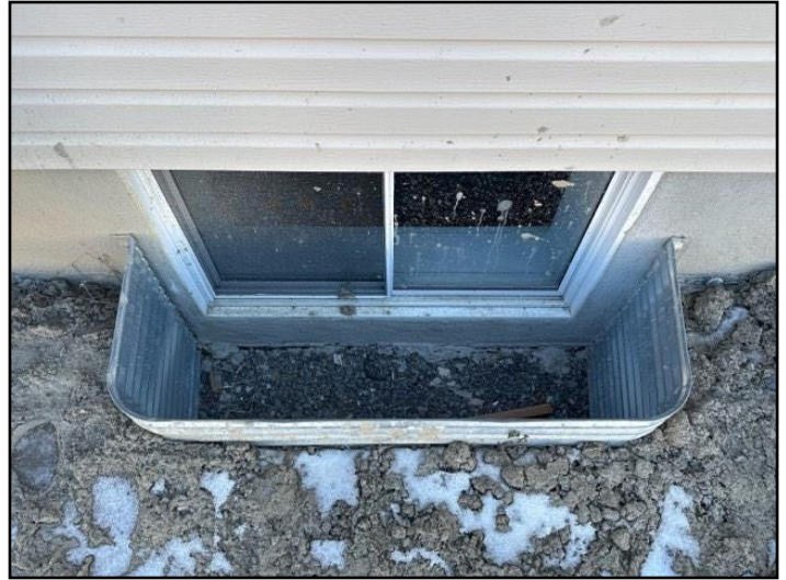
89. Clean window well
