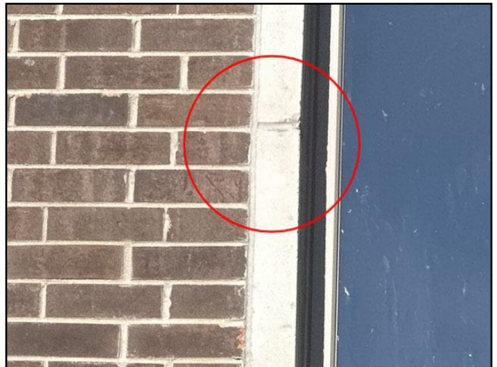
48. Masonry deterioration
