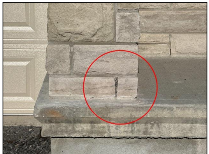
30. Masonry deterioration
