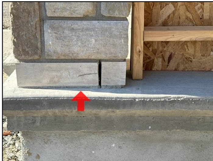
37. Masonry deterioration
