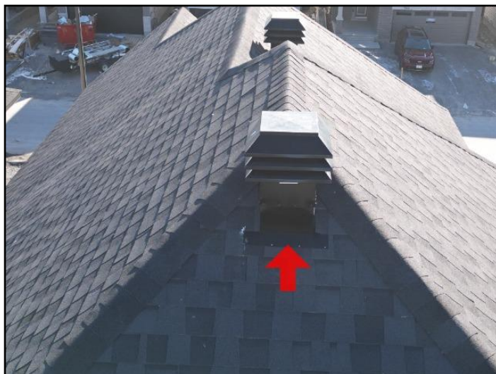
2. Exposed fasteners
