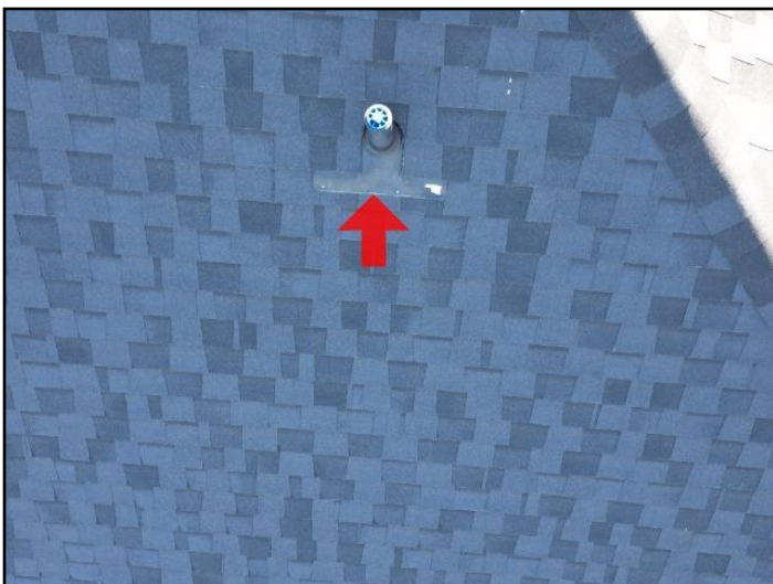
1. Exposed fasteners
