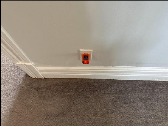
134. Ground needed for 3-slot outlet
