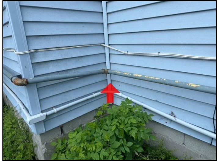
150. Inadequate support
