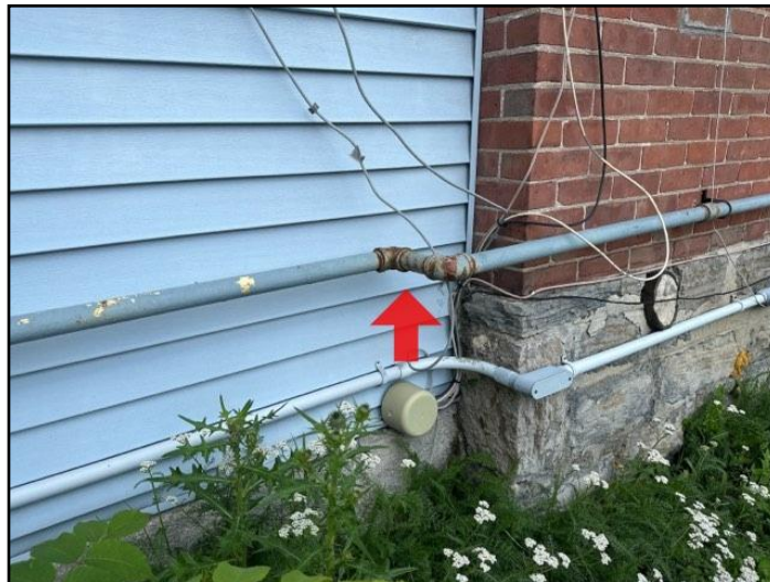
151. Inadequate support
