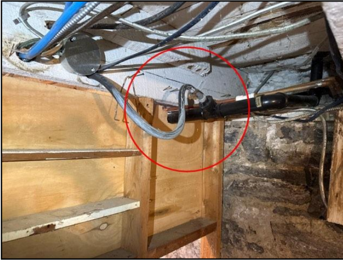
178. Dishwasher drain connections
