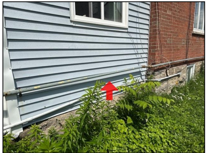
148. Inadequate support
