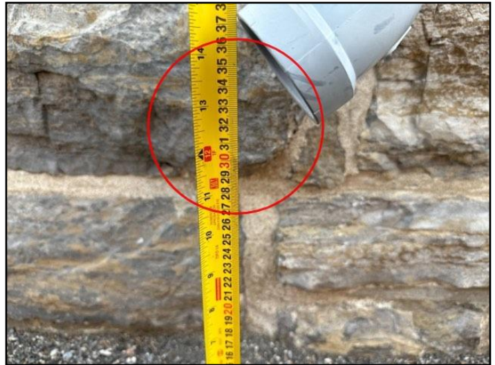
153. Rust, dirty, obstructed
