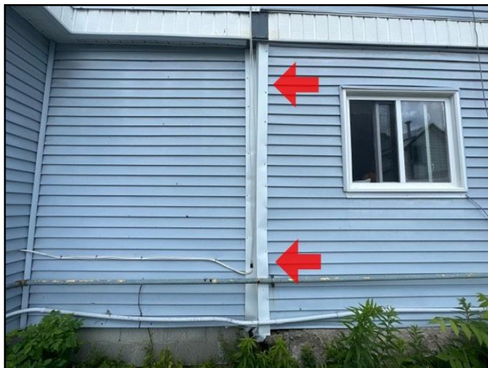
37. Mechanical damage
