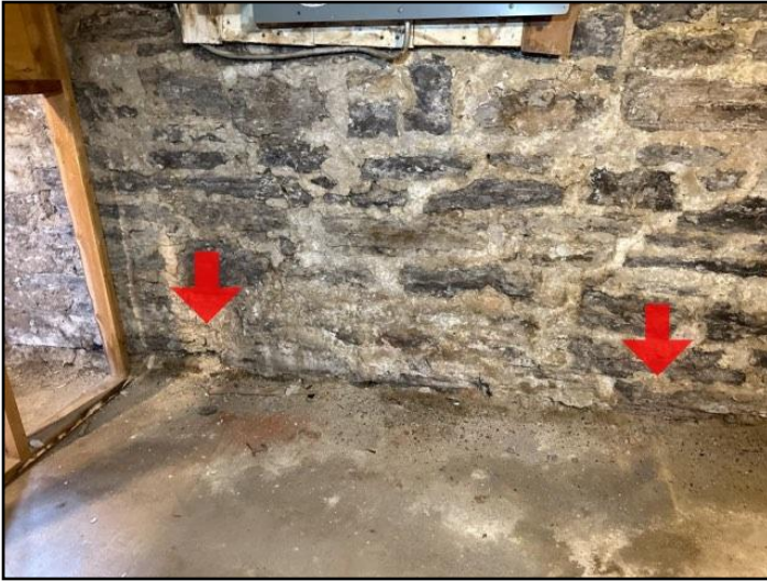
118. Mortar deteriorated or missing
