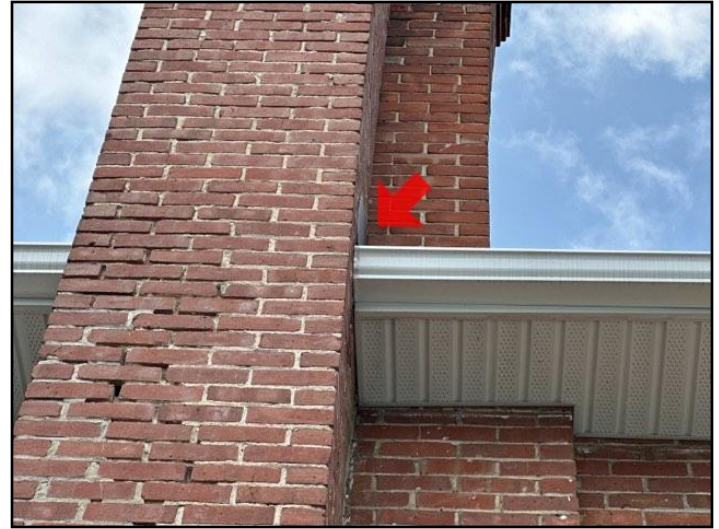
8. Kickout flashing - missing
