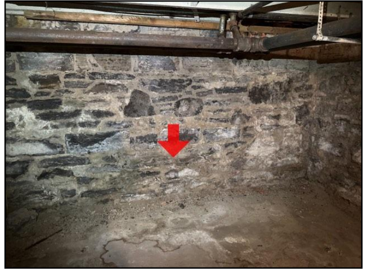
119. Mortar deteriorated or missing
