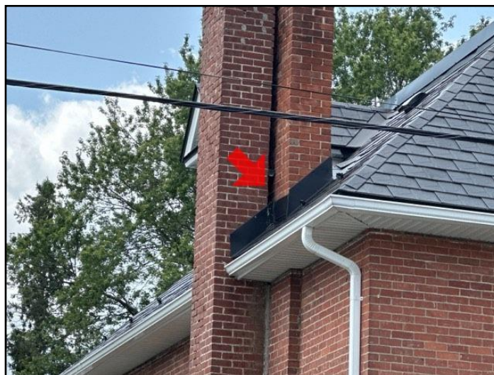
2. Not let into mortar joints
