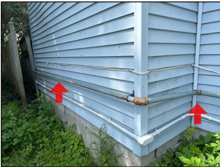
147. Inadequate support
