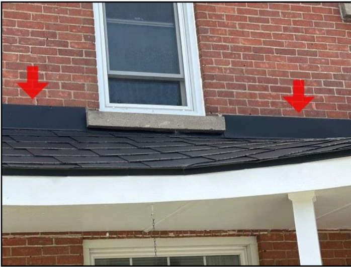
5. Not let into mortar joints
