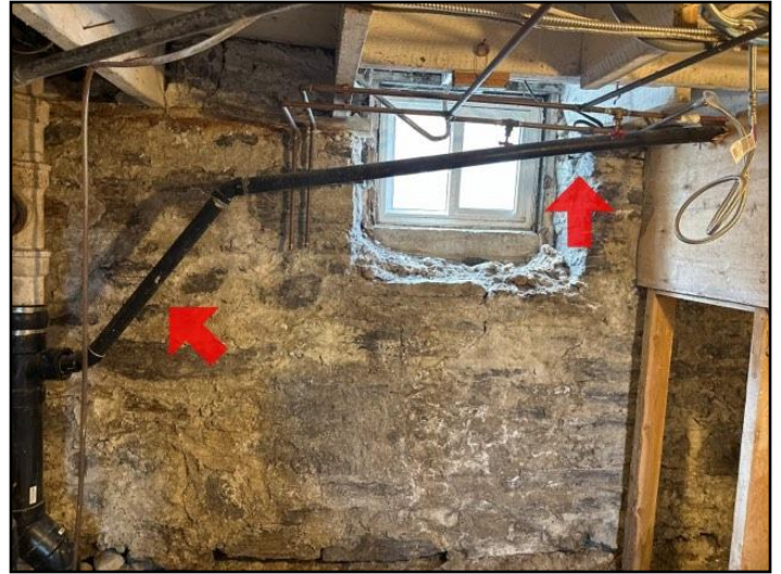
179. Dishwasher drain connections
