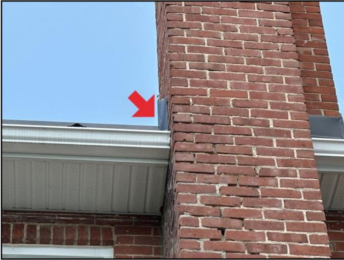
7. Kickout flashing - missing
