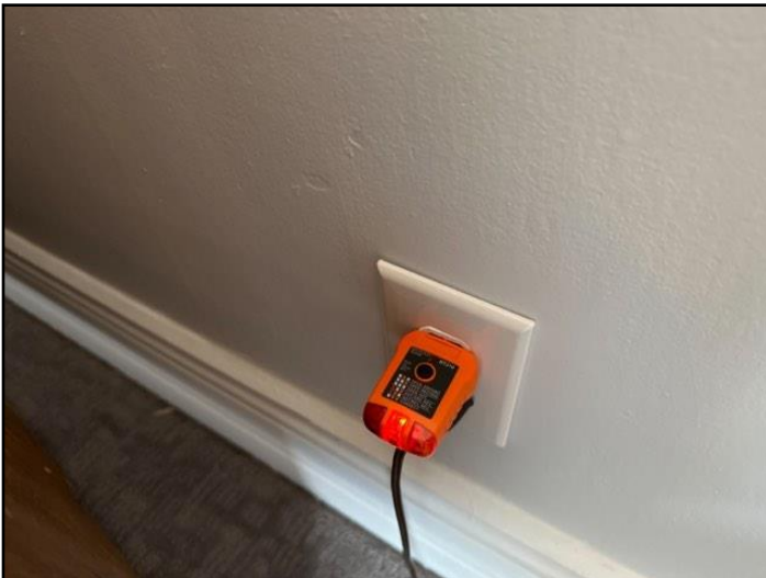
136. Ground needed for 3-slot outlet
