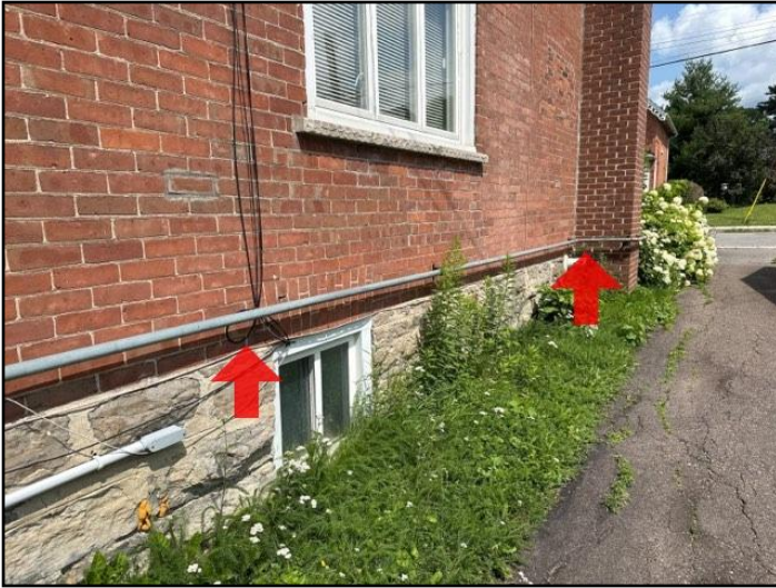
149. Inadequate support
