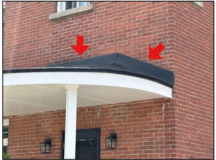
6. Not let into mortar joints
