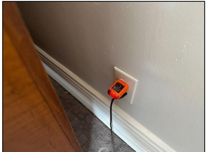
137. Ground needed for 3-slot outlet
