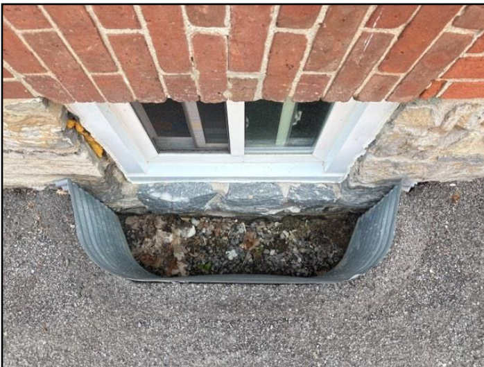
49. Clean window well
