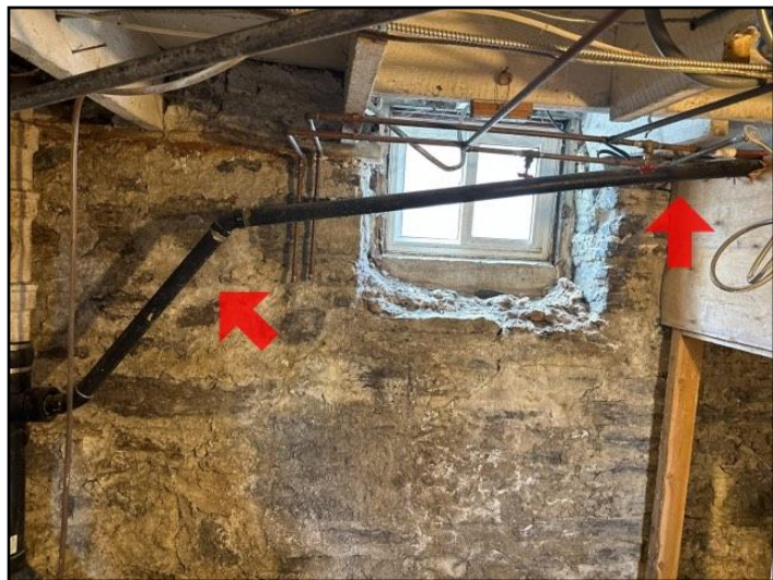
177. Poor slope
