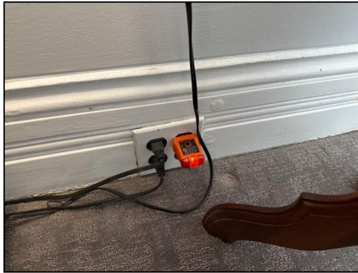
138. Ground needed for 3-slot outlet
