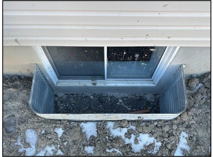
89. Clean window well
