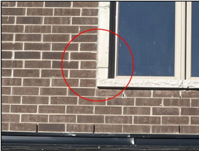
49. Masonry deterioration
