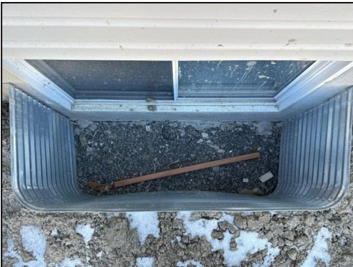
86. Remove all debris from window well.
