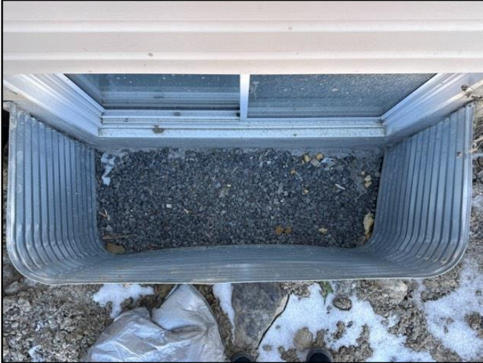
84. Remove all debris from window well.
