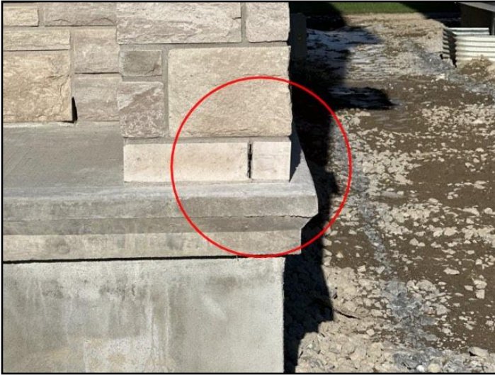
35. Masonry deterioration
