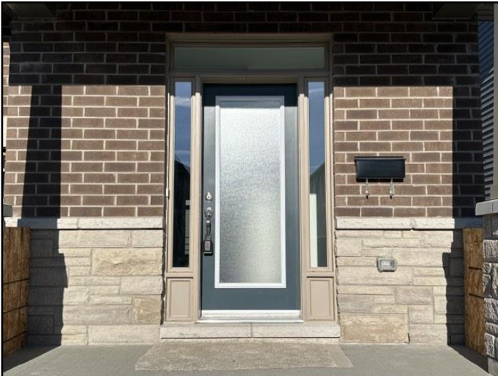
90. Damaged, cracked or loose
