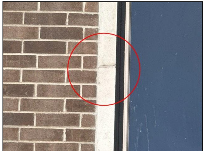
44. Masonry deterioration
