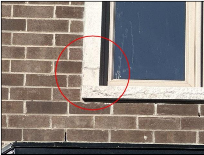
45. Masonry deterioration
