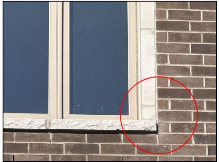
46. Masonry deterioration
