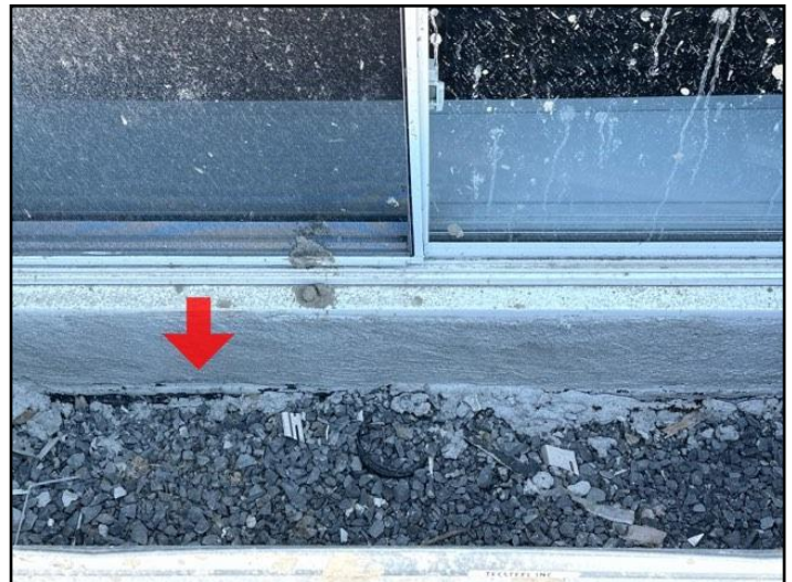
87. Remove all debris from window well.
