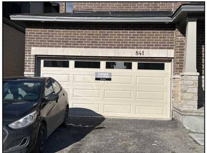
60. Debris on brick
