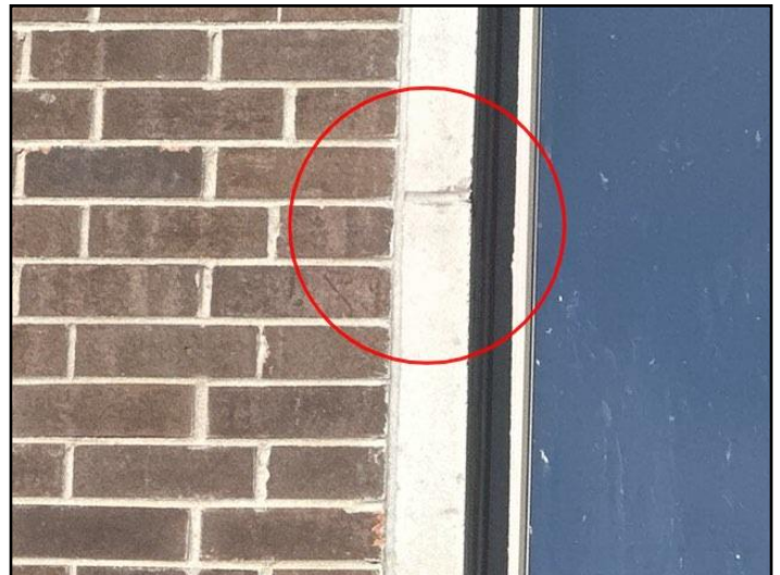
48. Masonry deterioration
