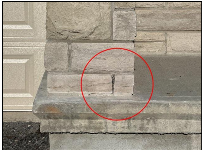
30. Masonry deterioration
