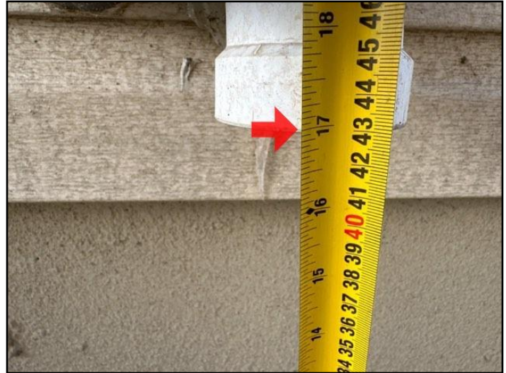
143. Clearance to grade
