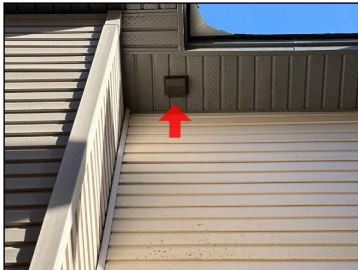
191. Clean dryer vent
