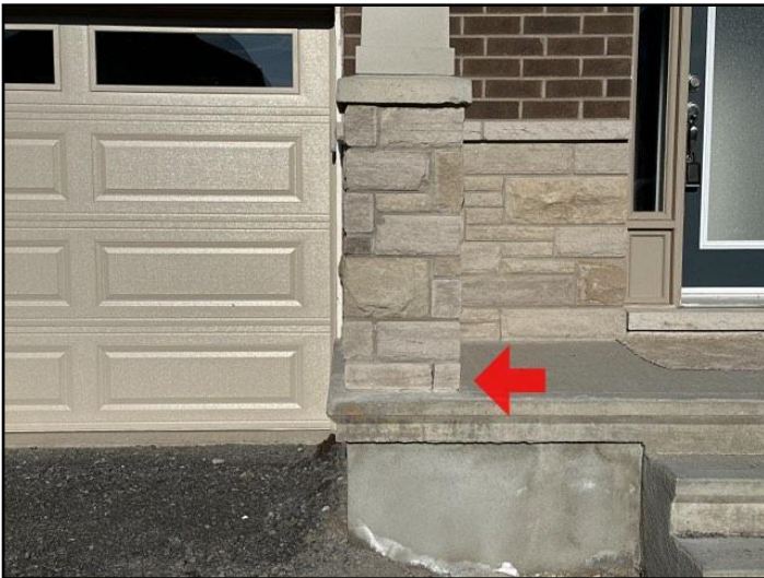
29. Masonry deterioration
