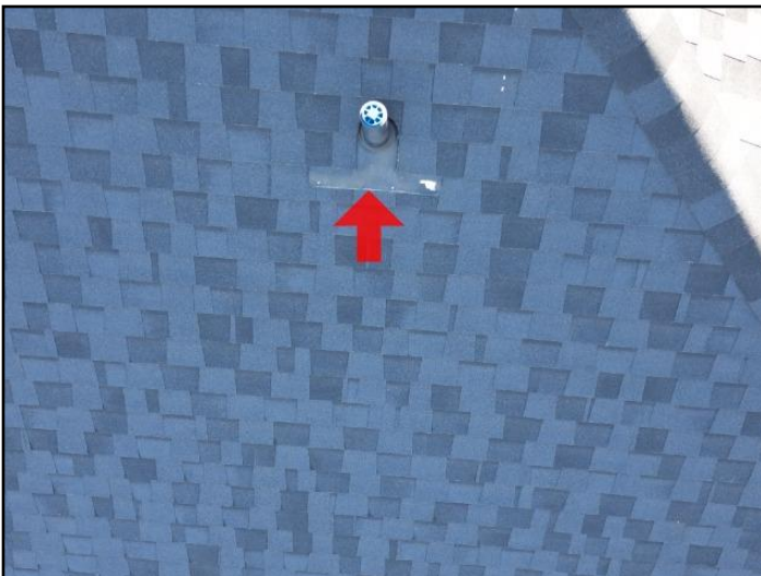
1. Exposed fasteners
