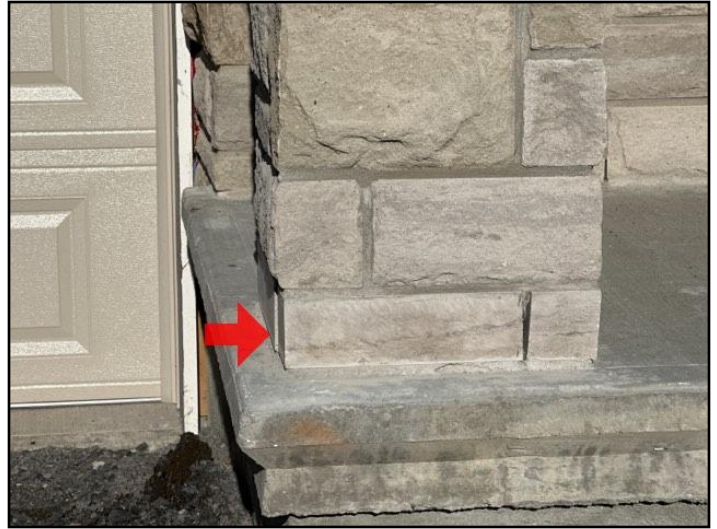
32. Masonry deterioration
