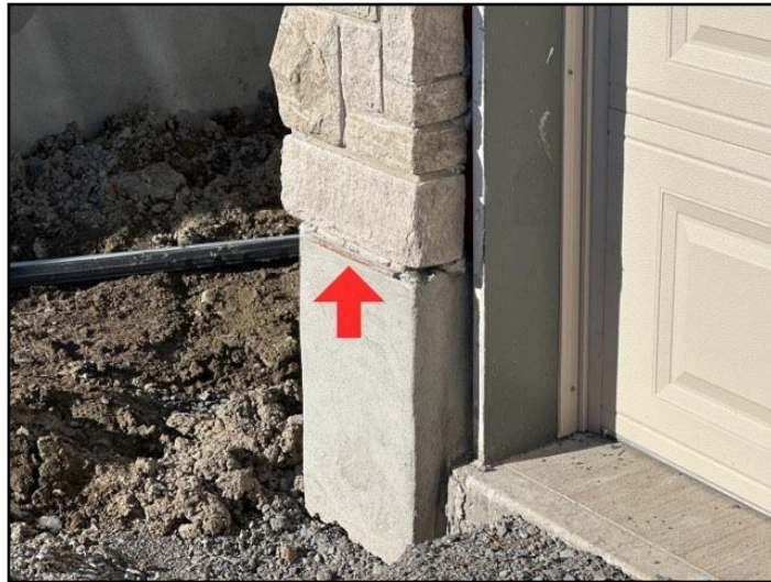
38. Masonry deterioration
