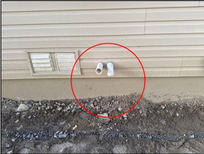
142. Clearance to grade
