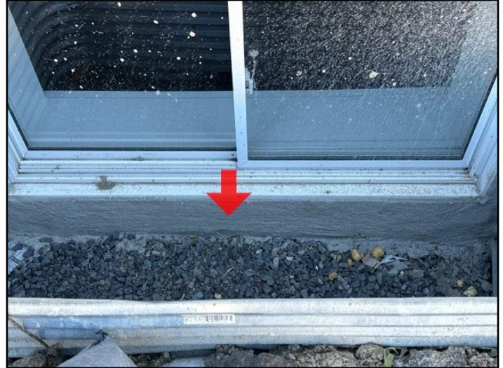
85. Remove all debris from window well.
