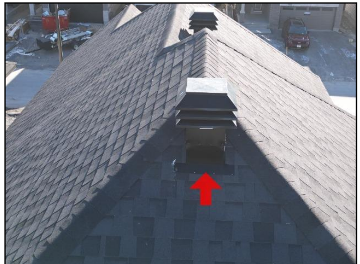
2. Exposed fasteners
