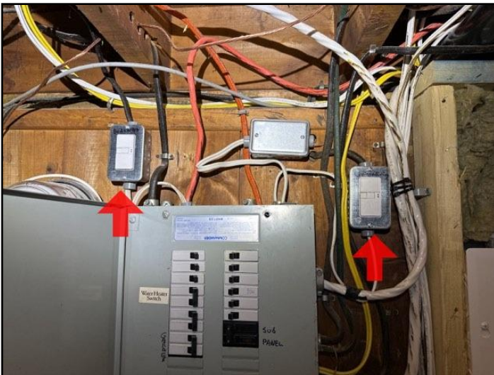
54. Ground needed for 3-slot outlet
