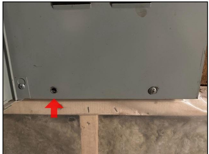
49. Panel screws can only be blunt end screws.
