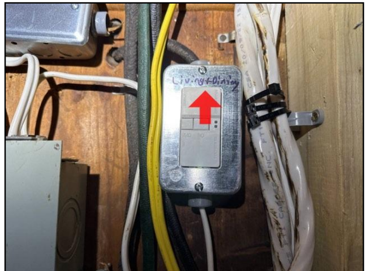
55. Ground needed for 3-slot outlet
