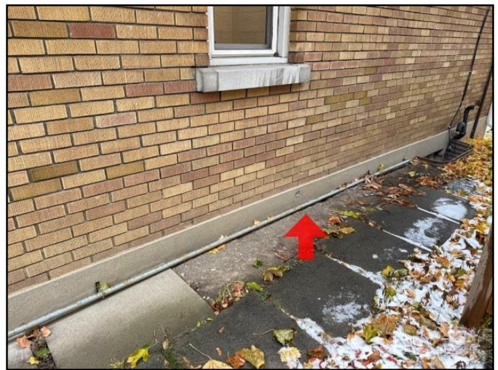
71. Inadequate support
