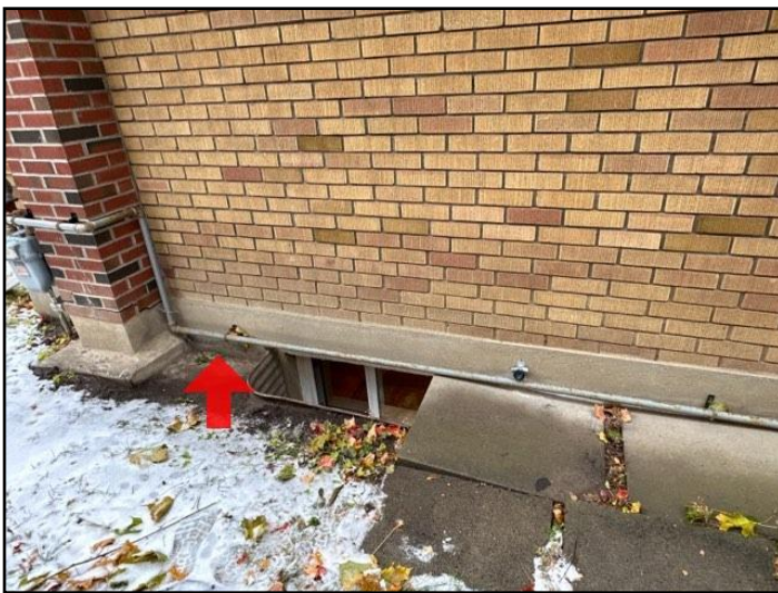
70. Inadequate support
