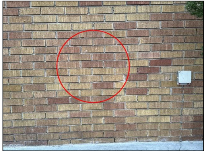
8. Mortar deterioration
