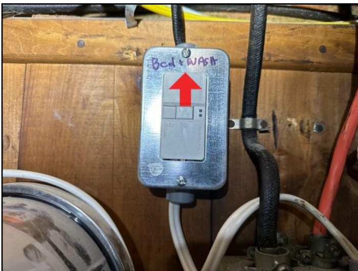
56. Ground needed for 3-slot outlet
