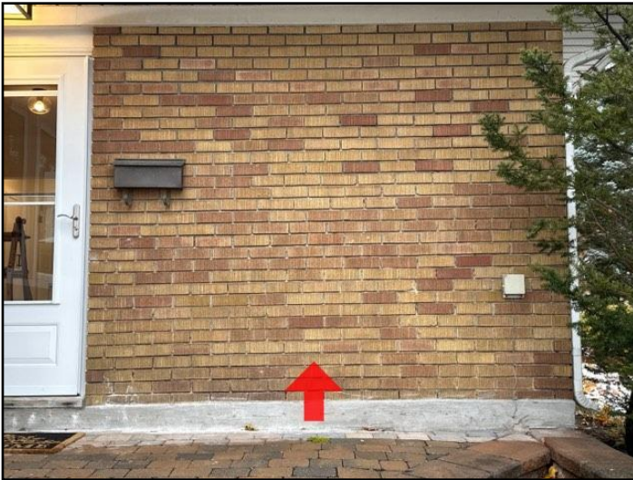
7. Mortar deterioration
