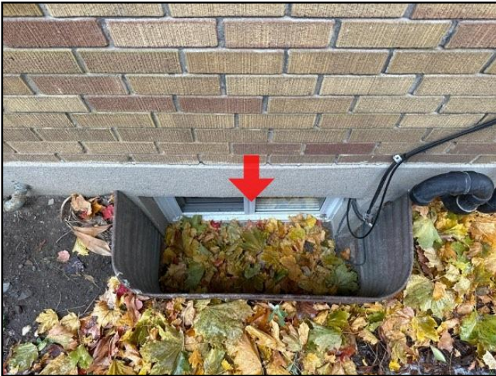
13. Clean window well
