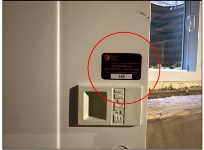
53. Modified or added wiring
