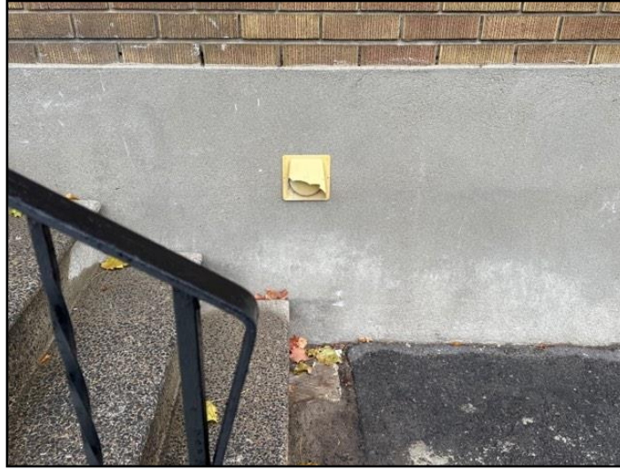
11. Cover damaged
