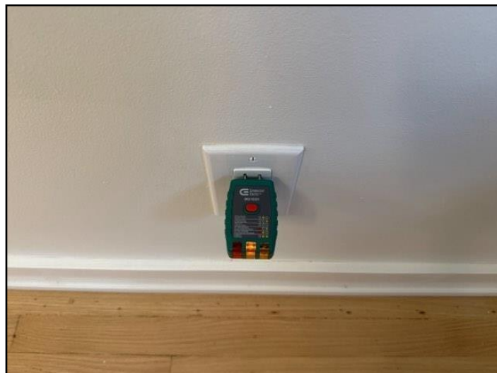
57. Ground needed for 3-slot outlet
