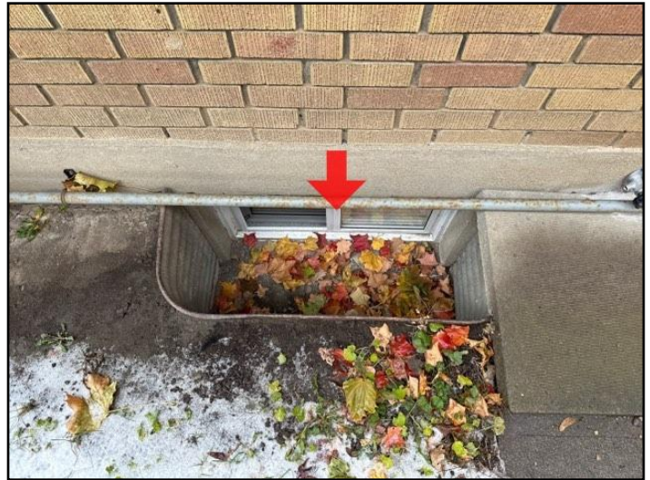
14. Clean window well
