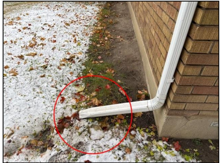
6. Should discharge 6 feet from building
