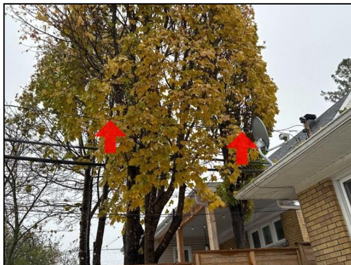
46. Branches / vines interfering with wires
