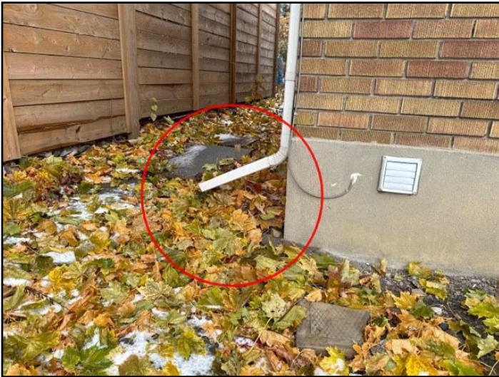
5. Should discharge 6 feet from building
