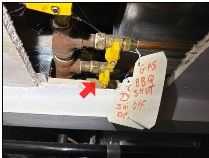
71. Gas line can not be modified by person othe...
