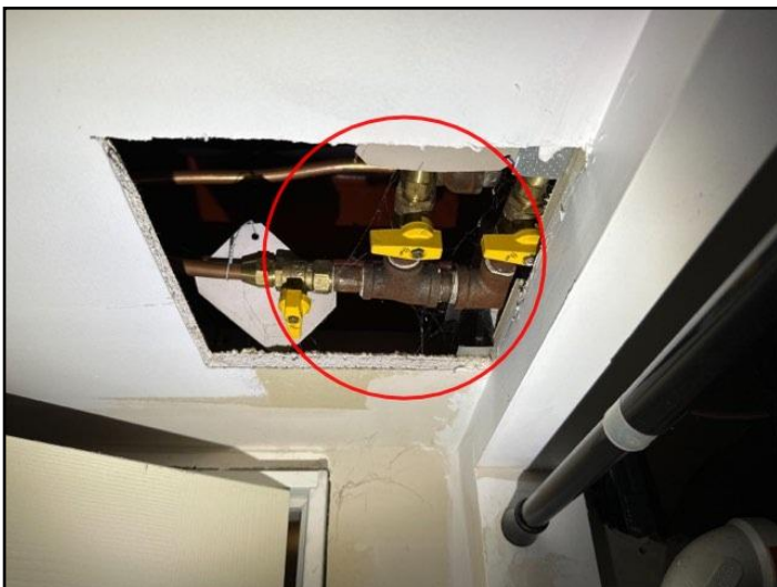
70. Gas line can not be modified by person othe...
