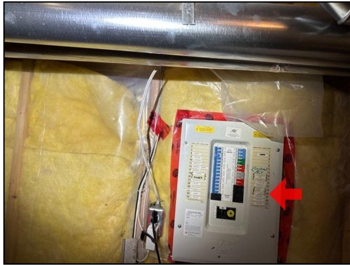
46. The house is equipped with a Federal Pacifi...
