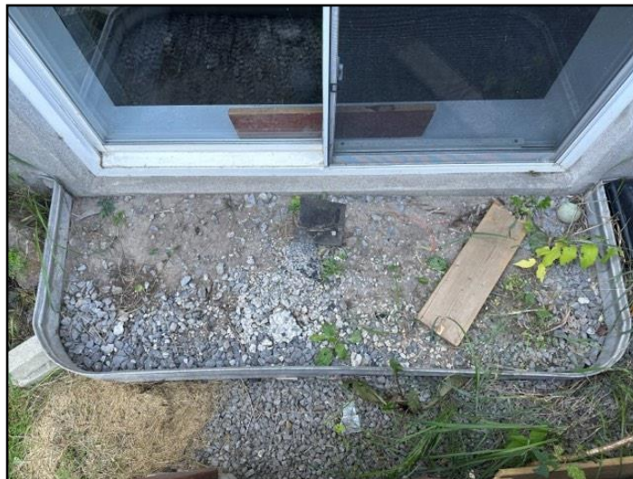
14. Remove all debris from window well.
