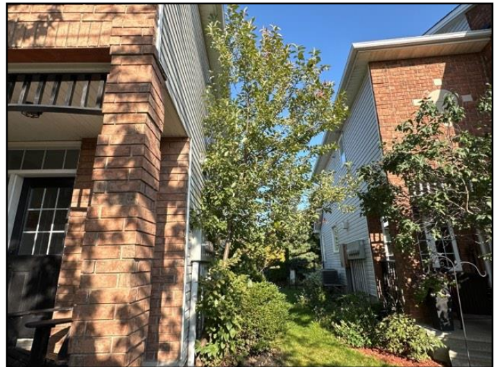
19. Trees or shrubs too close to building
