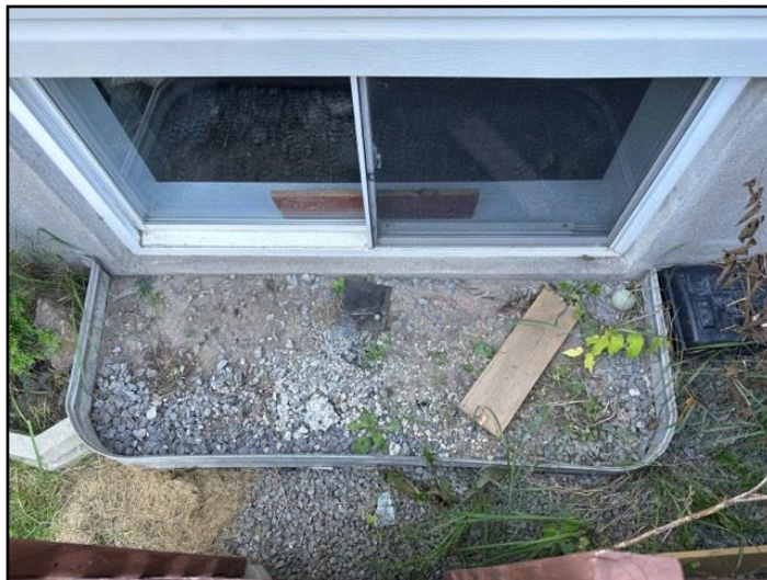
15. Clean window well
