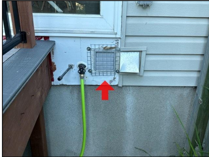
131. Clean dryer vent
